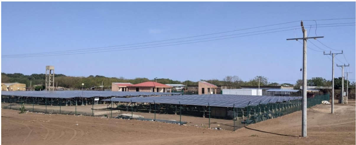
Fig. 16. A view of the PV MG infrastructure in Omorate, Dasanech district, Southern Ethiopia
