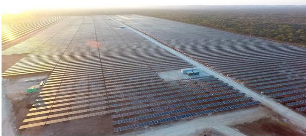
Fig. 25. Ngonye solar plants, in the Lusaka south multi facility economic zone
